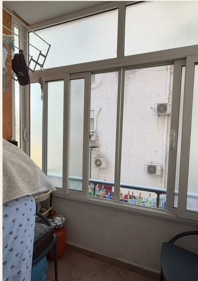
The enclosed balcony
